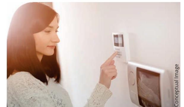
Video Intercom Facility
