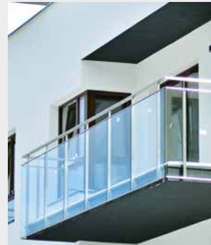
Balconies with skid resistant tile flooring and aluminium glass railings
