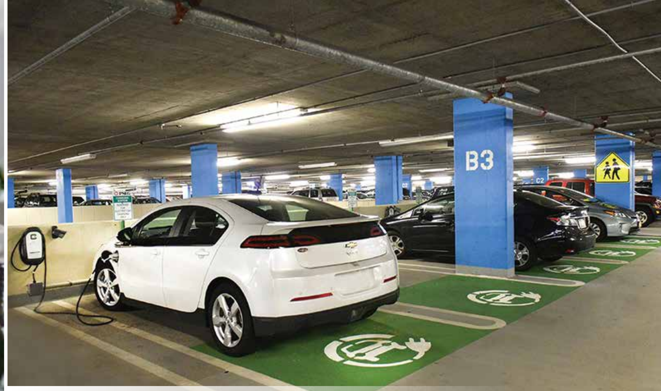
Full Car Park E.V. Ready
