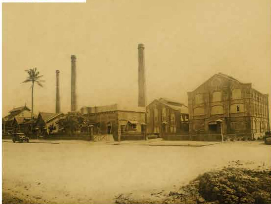
Pumping Station, Worli
