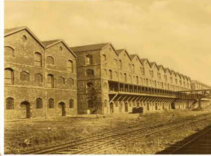
Mumbai Port Trust - Warehouse
