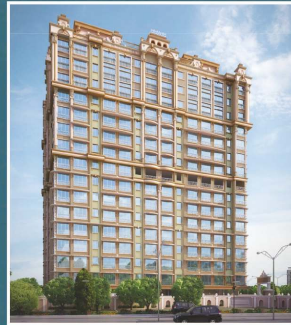
MILLIONAIRE HERITAGE, S. V. ROAD, ANDHERI (W)
